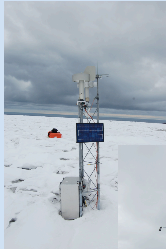
Measurements Before servicing
