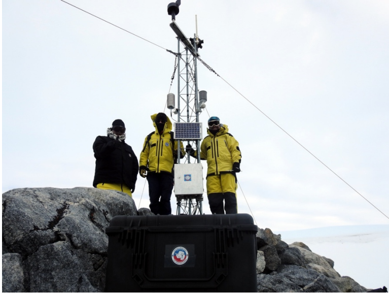
CDN after installation completed
