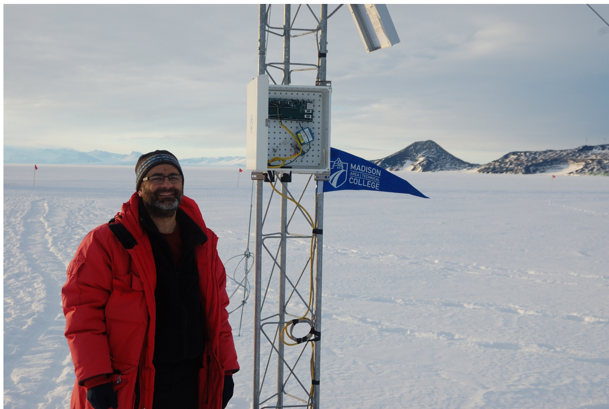
Prototype Madison College system installation at Willie Field.
