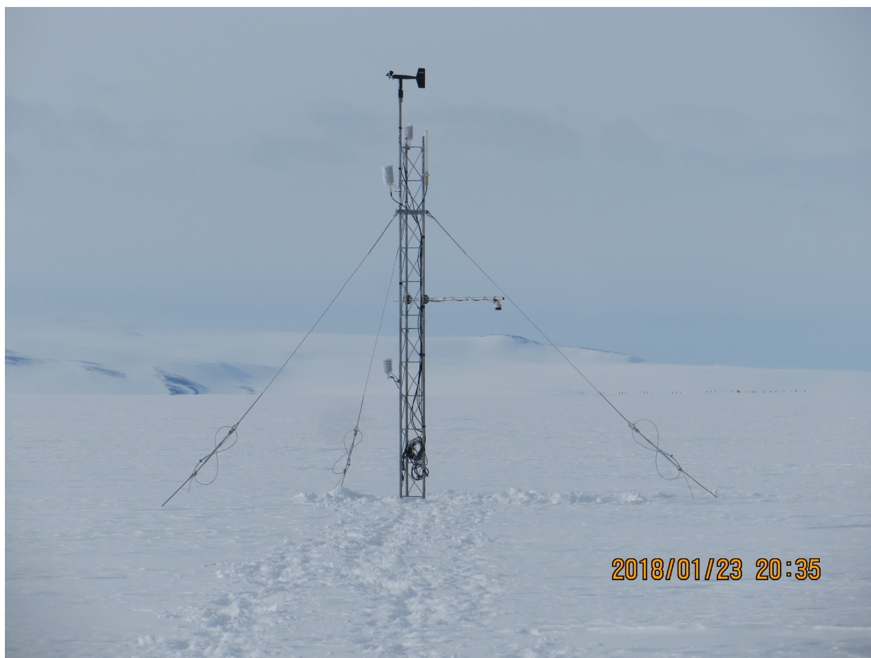
PHX with the power system and solar panel removed.
