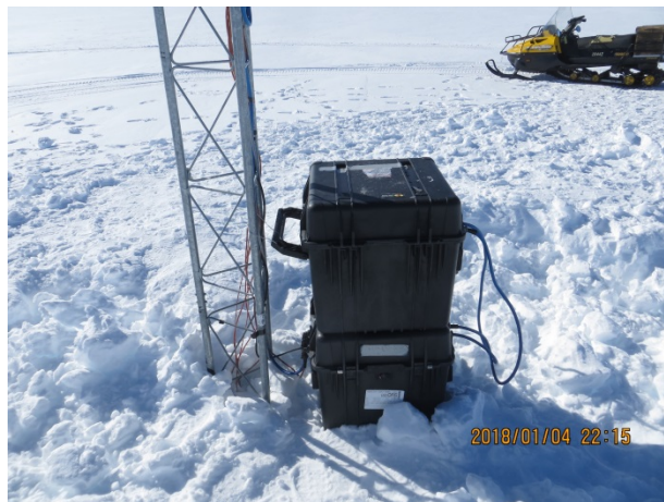
The stacked battery boxes
