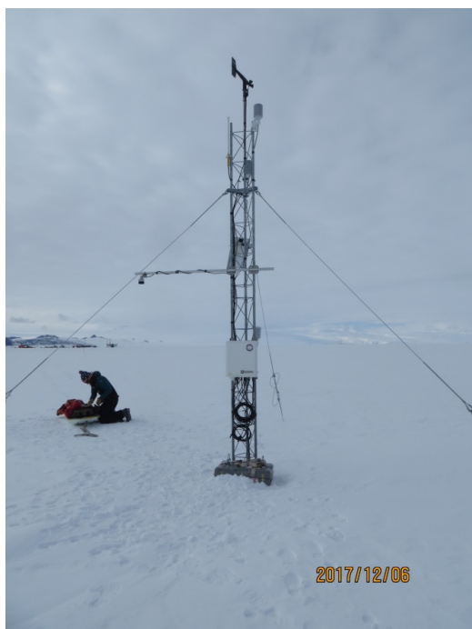
Phoenix AWS, after installing HMP
