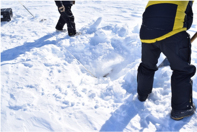
The shovel as a deadman
