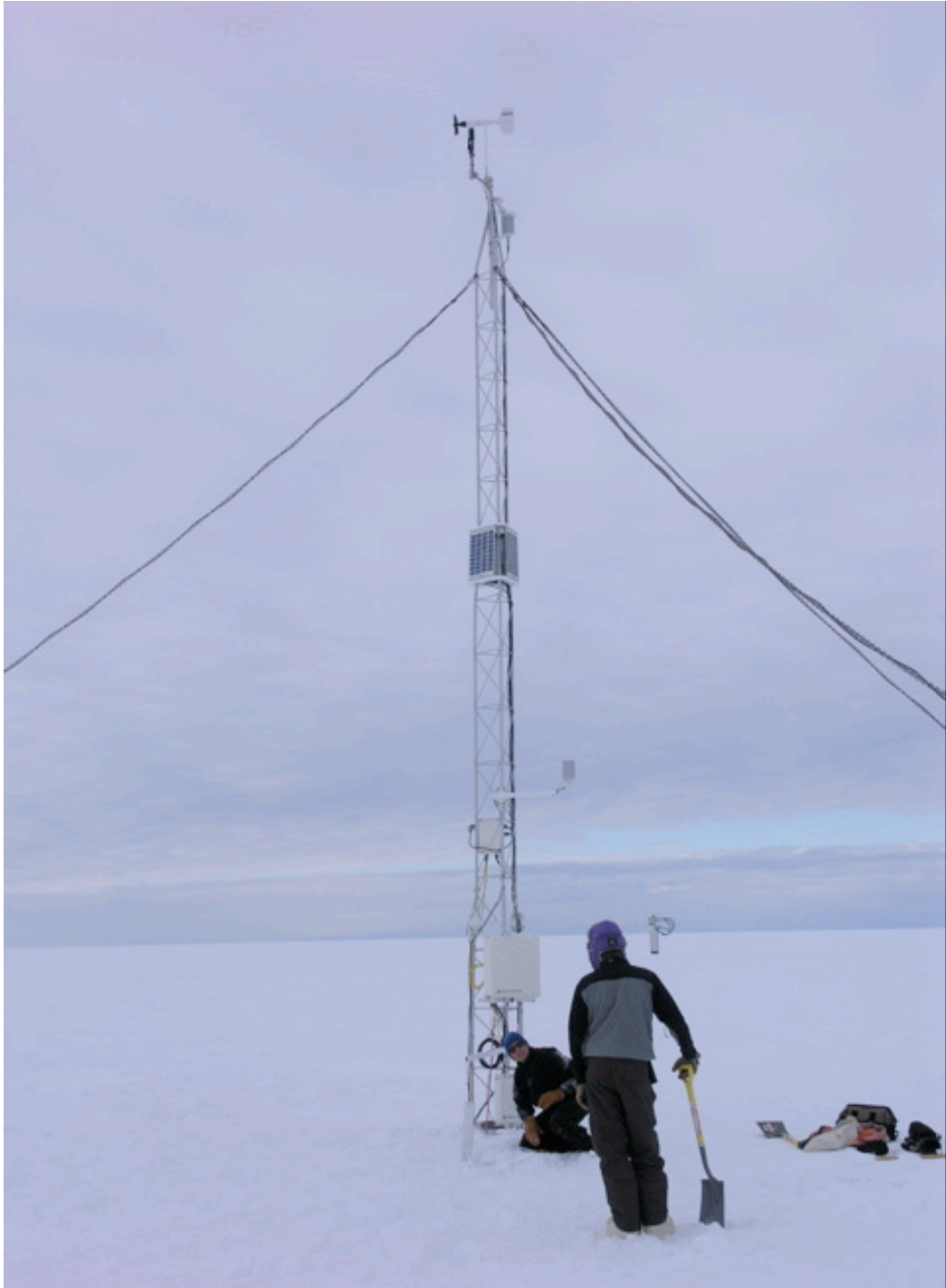
Figure 2: C-16 AWS - Mark II after repair of AWS.
