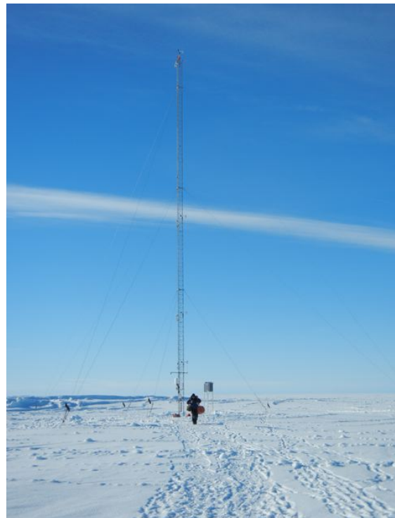
Figure 2. Tall Tower! Alexander AWS site after installation of several levels of instrumentation.
